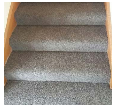
Waterfall Staircase Installation
